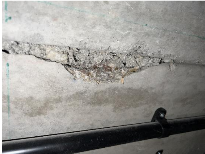
Image 7: Solid aggregates within panels
