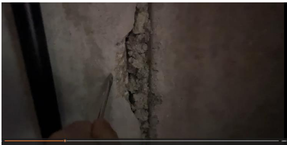
Image 4: Still from video of screwdriver test
