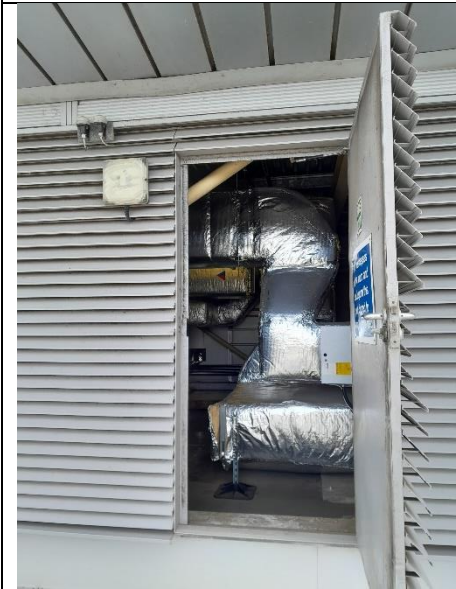
From roof back into plan room
