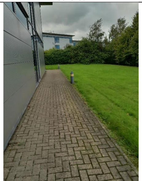
External routes clear with lighting
