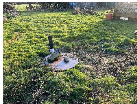
Photo 12: View of inspection cover of Klargester sewage treatment system
