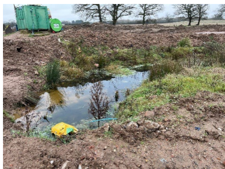
Photo 13: View of blocked land drainage due to tipping
