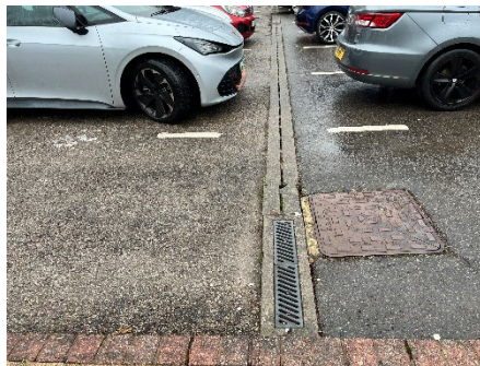
Photo 50: View of surface water drainage in front car park
