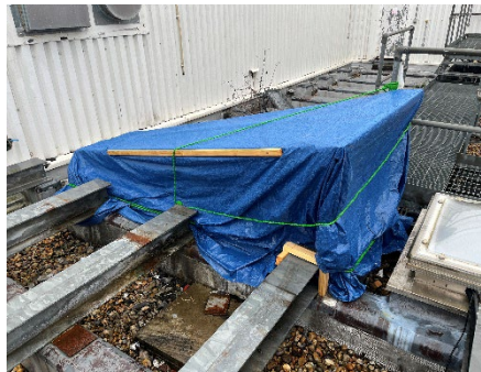
Photo 44: View of temporary repair to prevent water ingress through skylight on roof of Block B
