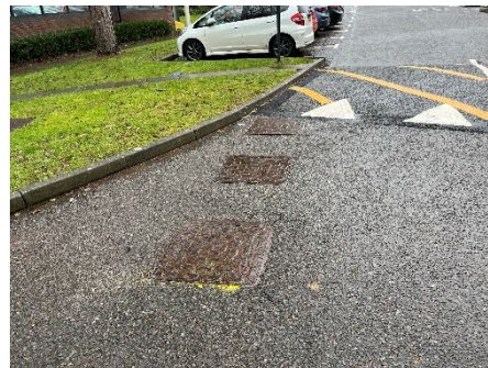
Photo 51: View of possible interceptor inspection covers on southwestern corner of Block A
