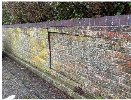
Photo 29: View of vehicle impact damage to southern boundary wall
