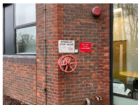
Photo 6: View of sprinkler cutoff valve (decommissioned) on eastern elevation
