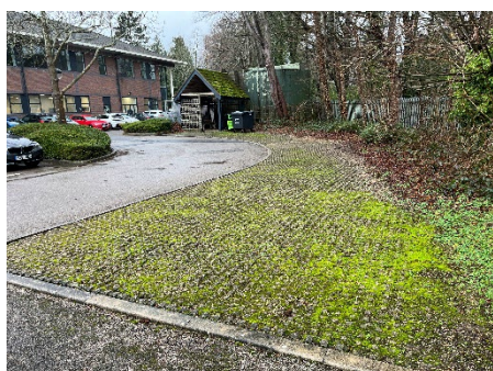
Photo 31: View of 'grasscrete' surfacing towards east of Block C
