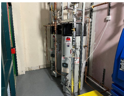
Photo 26: View of recently installed water heaters
