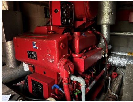
Photo 38: View of Cummins diesel powered generator (686 litre capacity) for the sprinkler pumps
