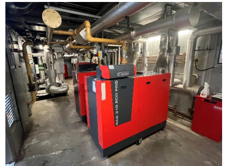
Photo 45: View of gas boilers in plant room on roof of Block B
