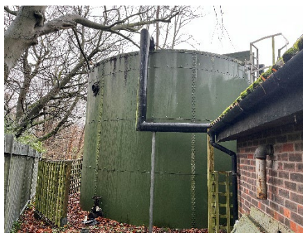
Photo 35: View of water sprinkler tank (installed 1987) understood to have been decommissioned
