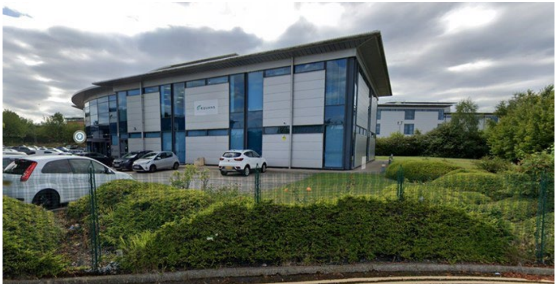
Photo 2: View South: Unit 3 [Google Streetview extract]
