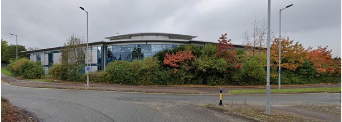
Photo 1: View west: Unit 2 [Google Streetview extract]
